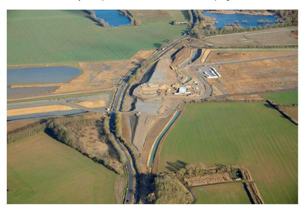
**Sections 4 & 5:** Work is underway to remove the temporary abutments which supported the bailey bridge at Swavesey junction. Construction of the permanent abutments next to the westbound carriageway at this location has started. This is in preparation for the installation of the first beams of the new bridge which will be built to the west of the current overbridge.
